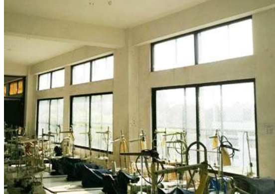
Figure: Sliding window used for ventilation
